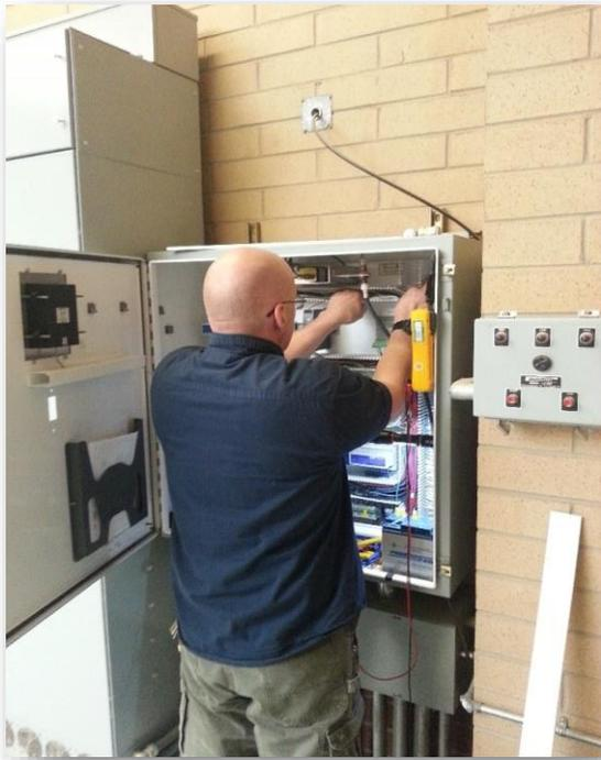
Repairs being made to the damaged U-111 RTU controller that was hit by lightning.
